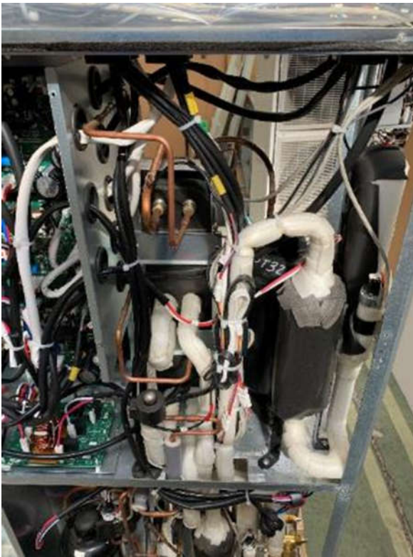
Before disconnecting and removing cables
